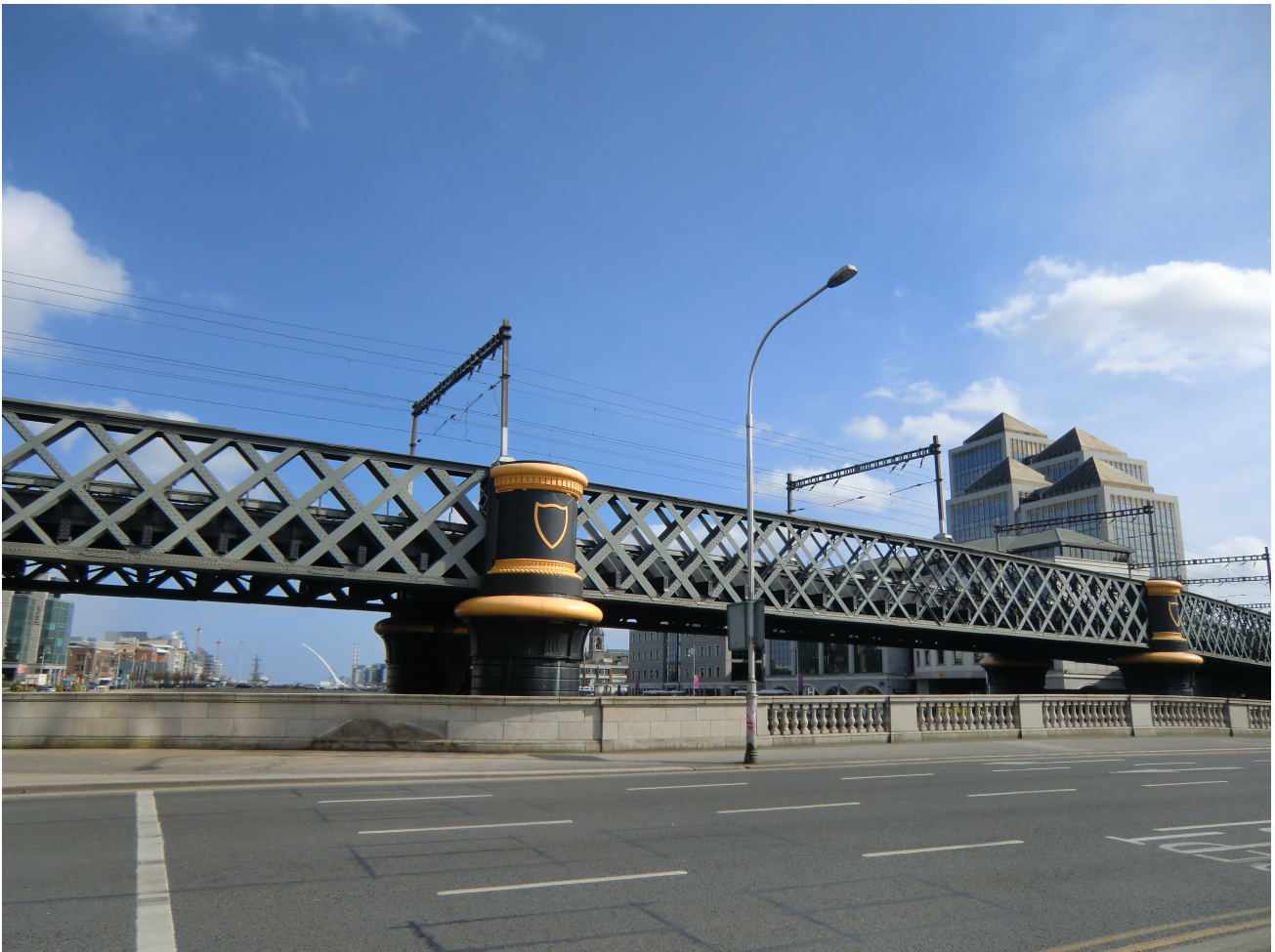
Dublin's Loophline Bridge
