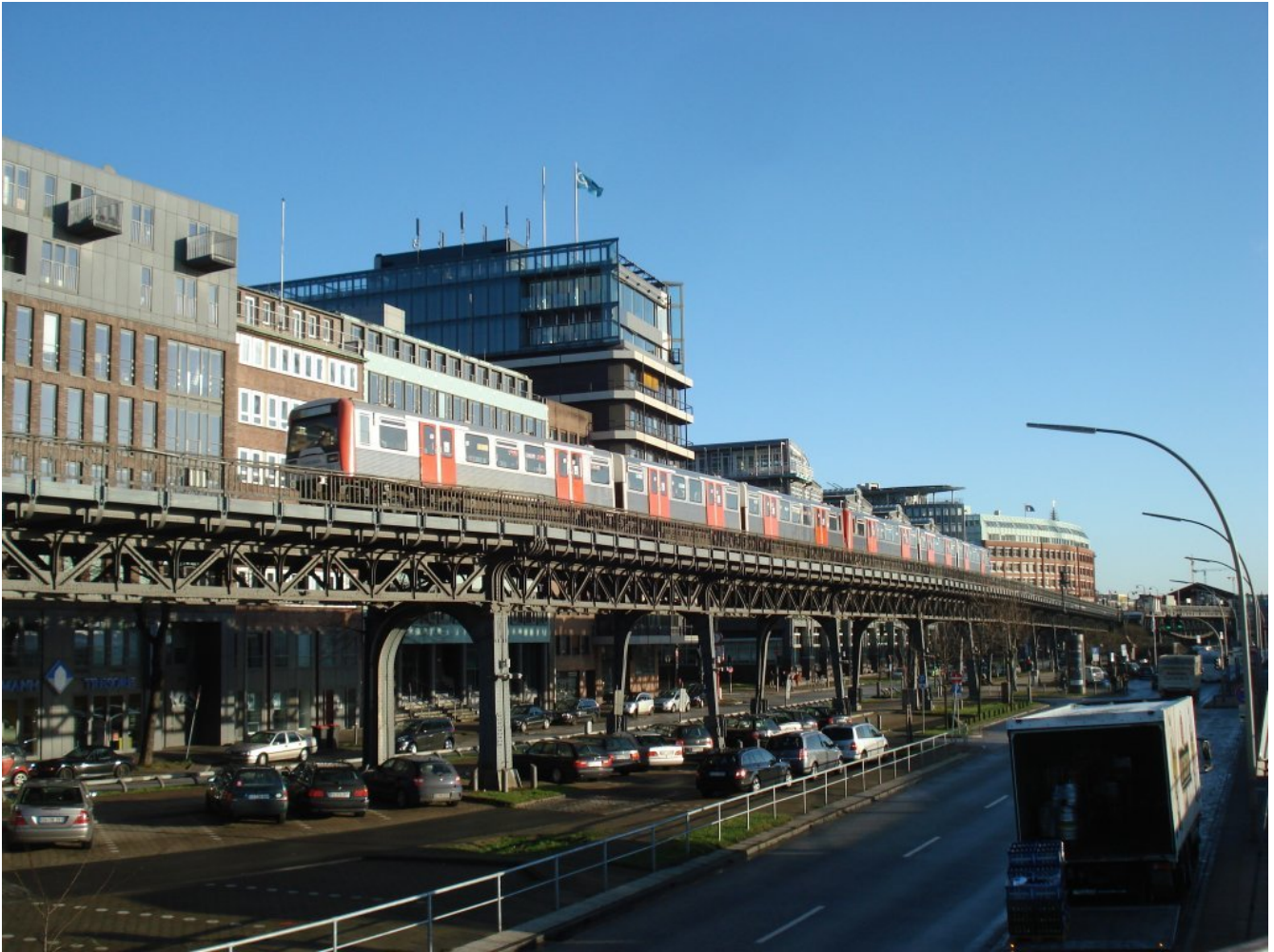
Elevated railway bridge in Hamburg, Germany
